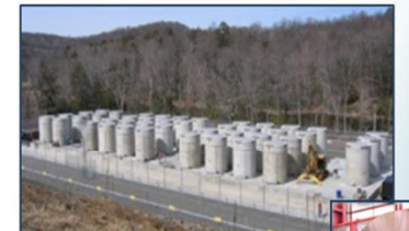
The fully-loaded pad will appear similar to the SNF storage pad shown above. The HLW Overpacks are designed for off-site transport via NAC's Storage and Transport Cask, pictured at right.
