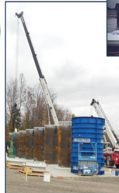
Upright liners with first form in place
