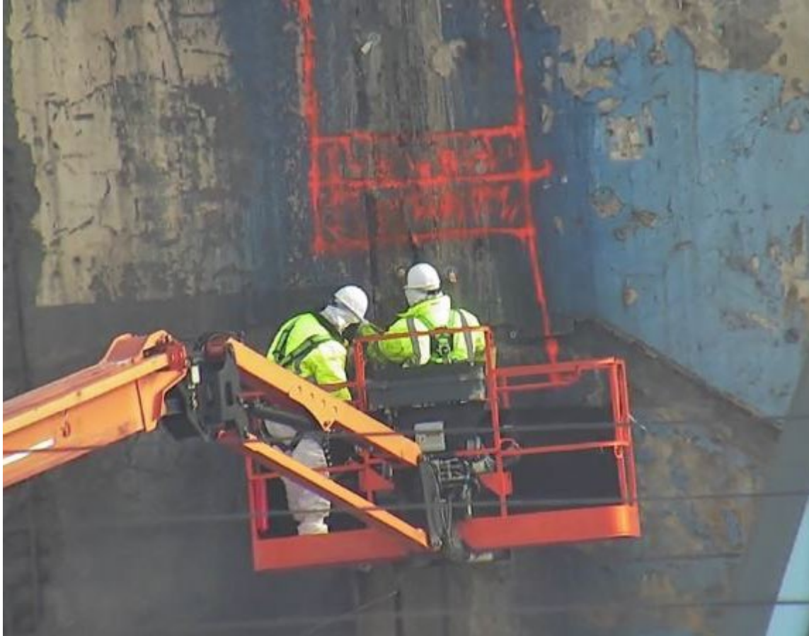
(Left) D&D operators mark demo areas on Off-Gas Cell (Right) Deconstructing OGC with hydraulic hammer
