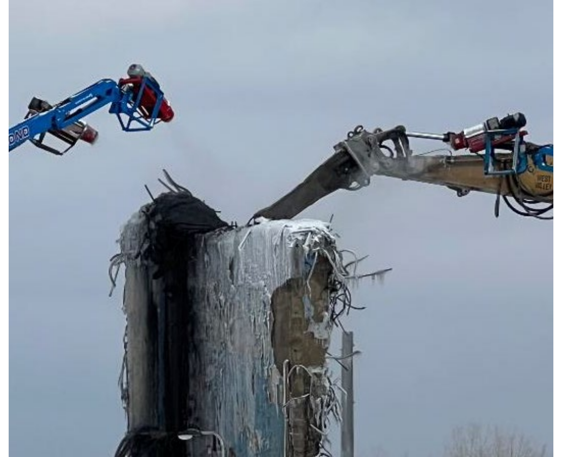
(Left) D&D operators mark demo areas on Off-Gas Cell (Right) Deconstructing OGC with hydraulic hammer
