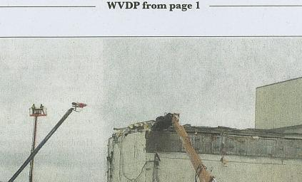
Heavy equipment is used to remove the roof of the Vitrification Facility at the West Valley Demonstration Project.
