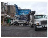
A pumper truck is used to place grout into the general purpose cell of the main plant process building at the West Valley Demonstration Project. The grout will provide structural stability to allow heavy demolition equipment to drive over the below grade rooms, while the main plant process building is being demolished.
