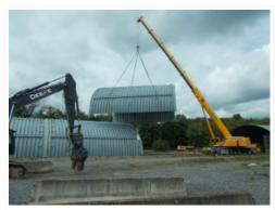
A large crane is used to relocate sections of the CPC-WSA to an area where they can be safely demolished.
