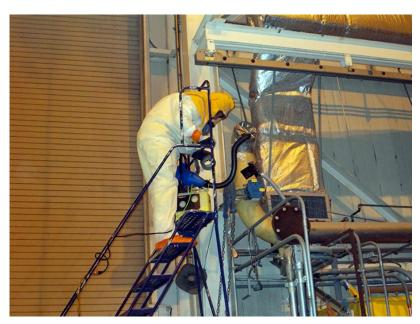
An operator inside the former fuel receiving and storage facility at the West Valley Demonstration Project Site pumps a fogging agent inside a pipe to fix suspected contamination. This work was part of deactivating the building for eventual demolition.
