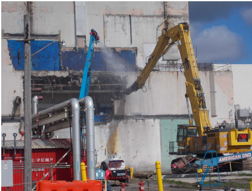
Main Plant deconstruction moves onto the Upper Warm Aisle
