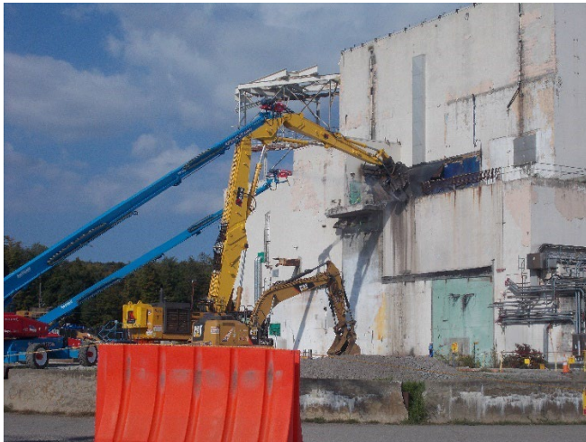
Main Plant deconstruction starts on with the Solvent Storage Terrace
