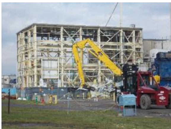
Load-In Facility demolition
