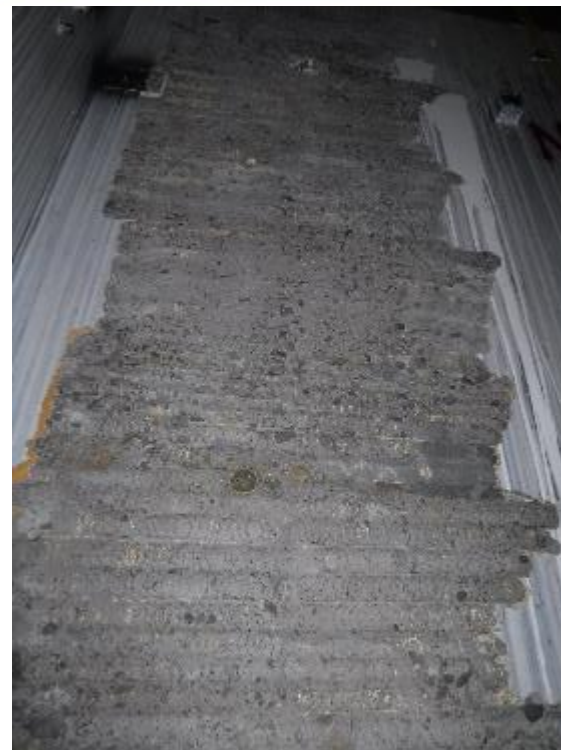
PPC-S wall 'scabbled' after using Nitrocision (November 2021)
