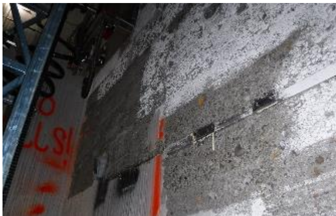
PPC-S wall 'scabbled' after using Nitrocision (November 2021)
