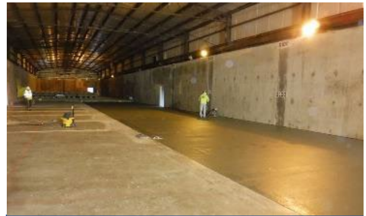
New concrete floor inside Drum Cell
