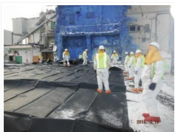
Workers at the West Valley Demonstration Project pull and smooth out the polyethylene weather protective cover over the vitrification facility concrete slab.
